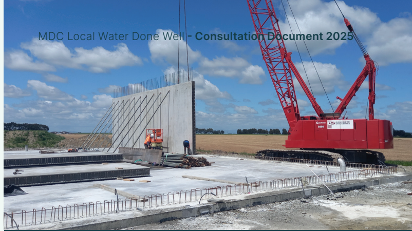
Stanway-Halcombe Water Reservoir
