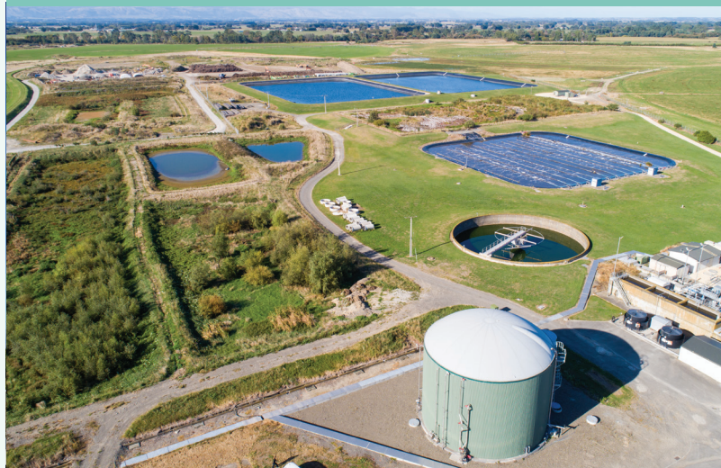
MDC Wastewater Treatment Plant
