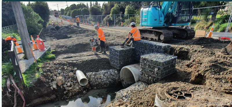
Stormwater upgrades Rongotea
