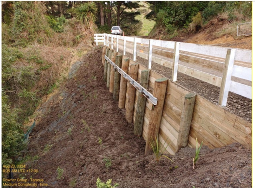
Maunga Road retaining wall completed.
