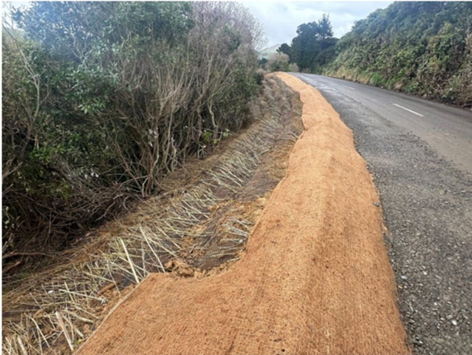
Tourere Road – High specified willow brush retaining wall completed in August.
