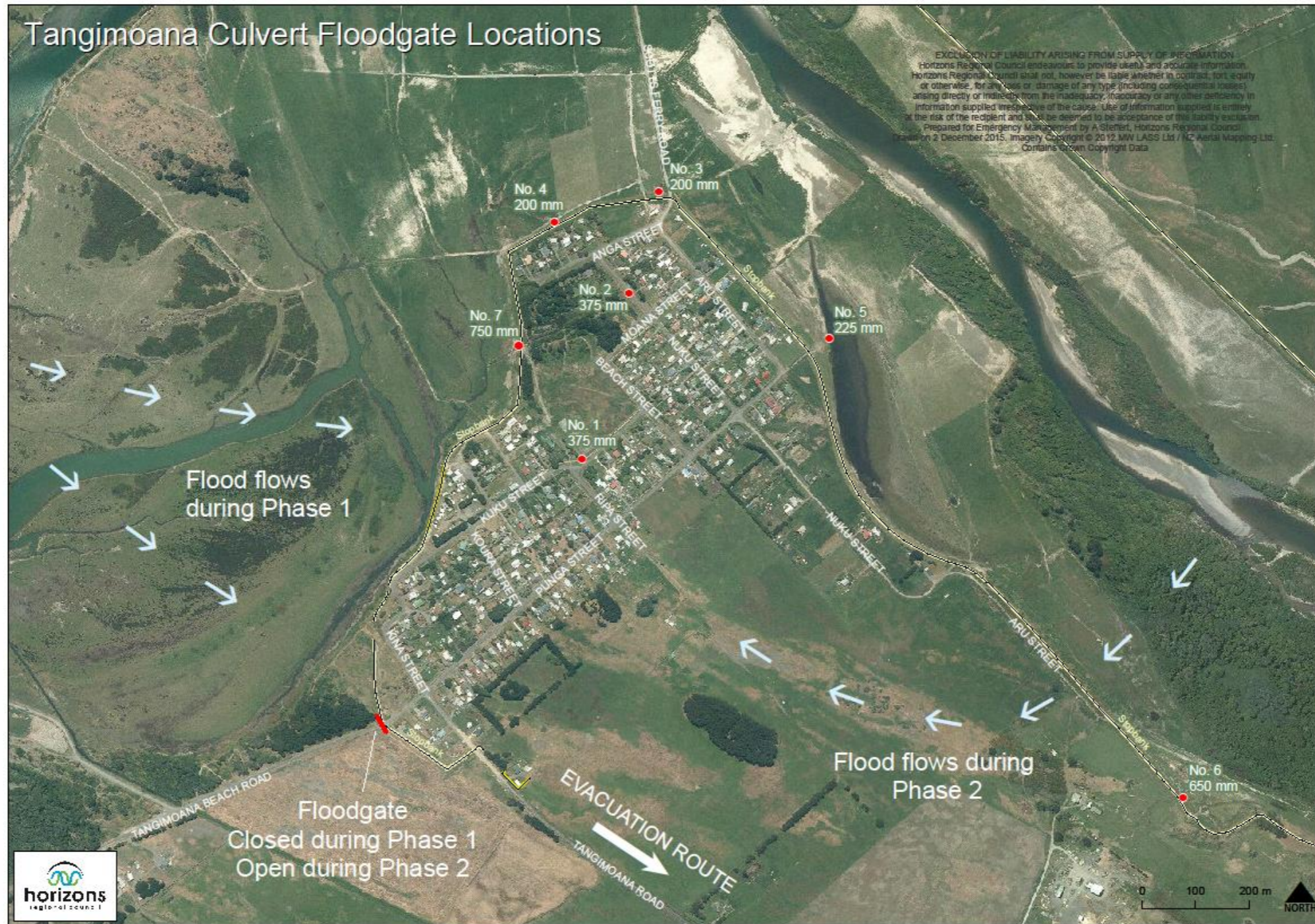
Figure 1: Culvert Flapgate Locations
