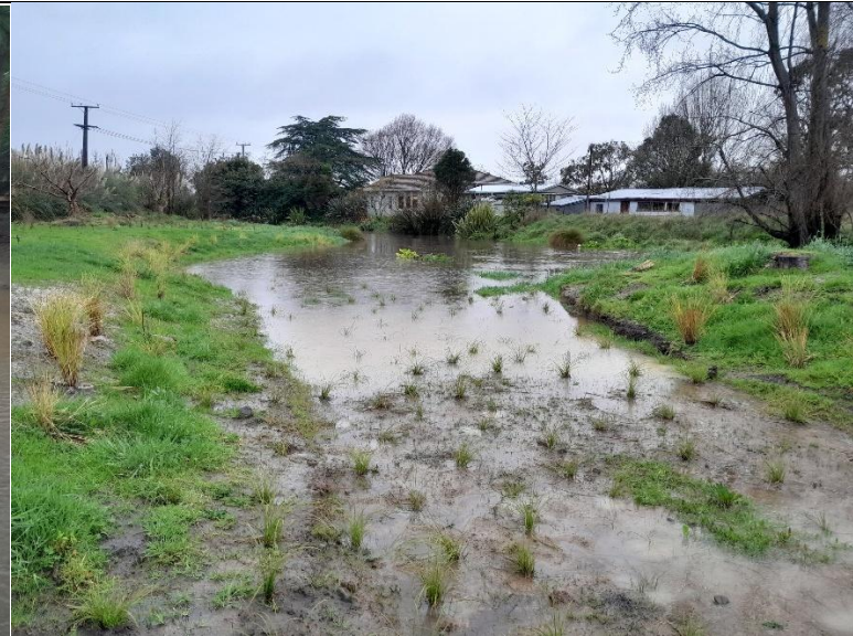
New plantings in reconstructed spillway survived first flood No plants washed out – Wetland site
