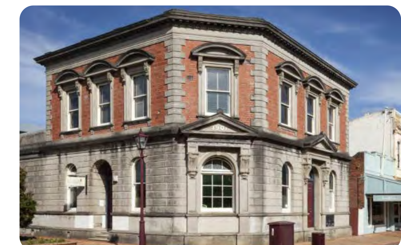
Keeping it real with existing features being supported to be kept
