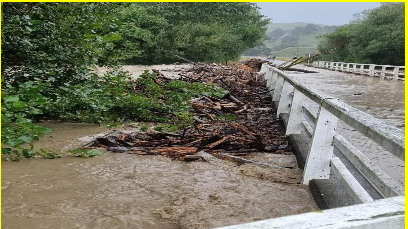
Coulters Line Bridge 2023
