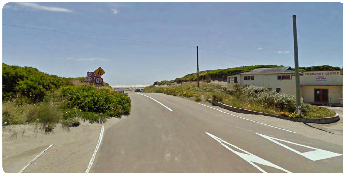
Sand blows off the beach onto the street
