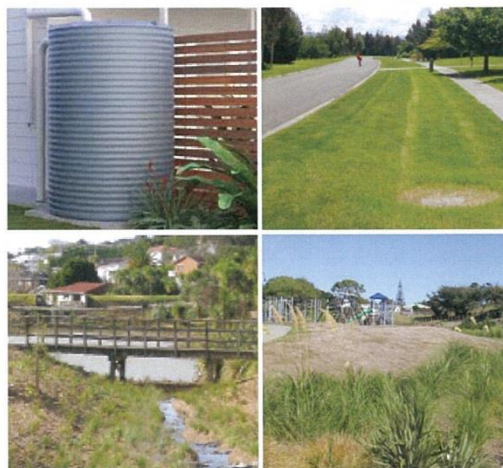
Examples show the network process, clockwise from top left - collection of stormwater at source - to rainwater tanks from roofs and to swales from roads, the direction of that runoff to a filtering area and then its discharge finally through a re-vegetated local stream to the receiving water course
