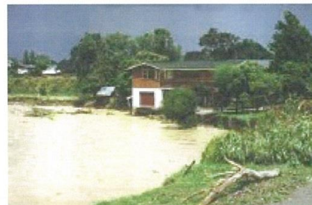
The Feilding town sits on a flood plain. It is important to plan new development to recognise hazards and to minimise the extent to which new development may exacerbate them
