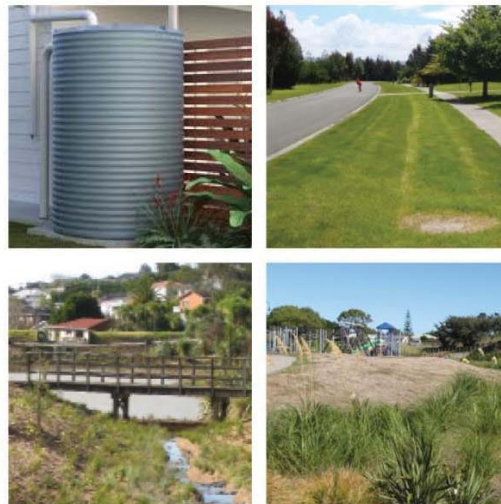
Examples show the network process - collection of stormwater at source - to rainwater tanks from roofs and to swales from roads, the direction of that runoff to a filtering area and then its discharge finally through a re-vegetated local stream to the receiving water course.
