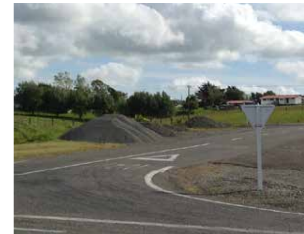
Establish appropriate maintenance protocols / weed control
