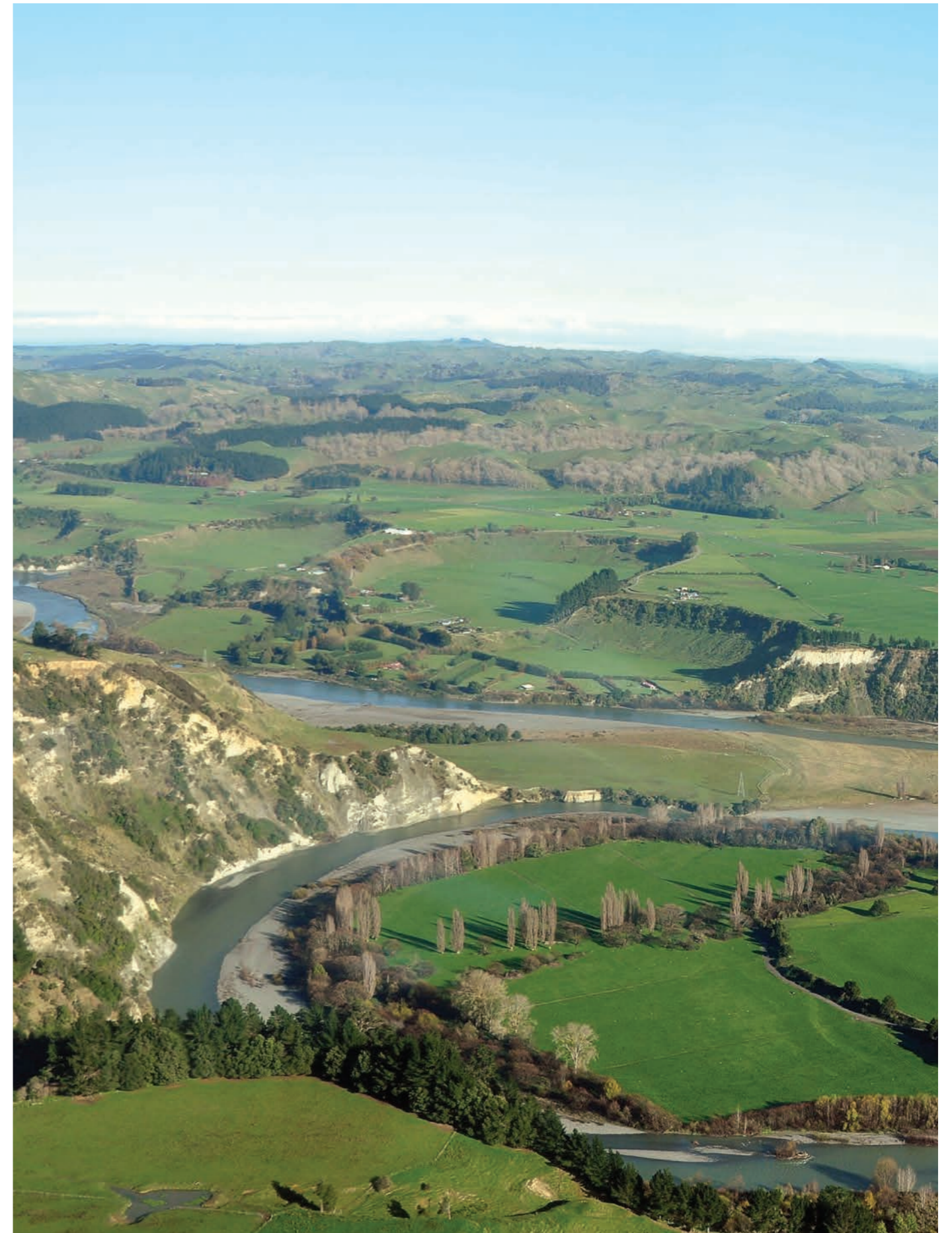
Rangitikei Photo 3- High voltage Bunnythorpe to Ongarue A (110Kv) transmission line crossing the Rangitikei River
