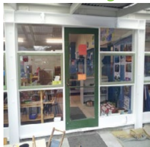
The two examples of external strengthening above contrast. The poor example (left) has cross braces (painted green) that run diagonally counter to the building's modulation. The good example (right) has a portal type bracing that fits with the door and window frame proportions and is painted the same principal white colour to de-emphasise it.
