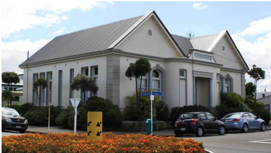
Feilding Community Centre, 21 Stafford Street (constructed 1910)
