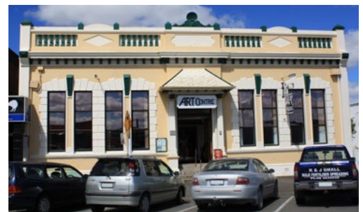
Photograph of Art Centre, 35 Kimbolton Road (formerly Rangitikei Club) - constructed 1911
