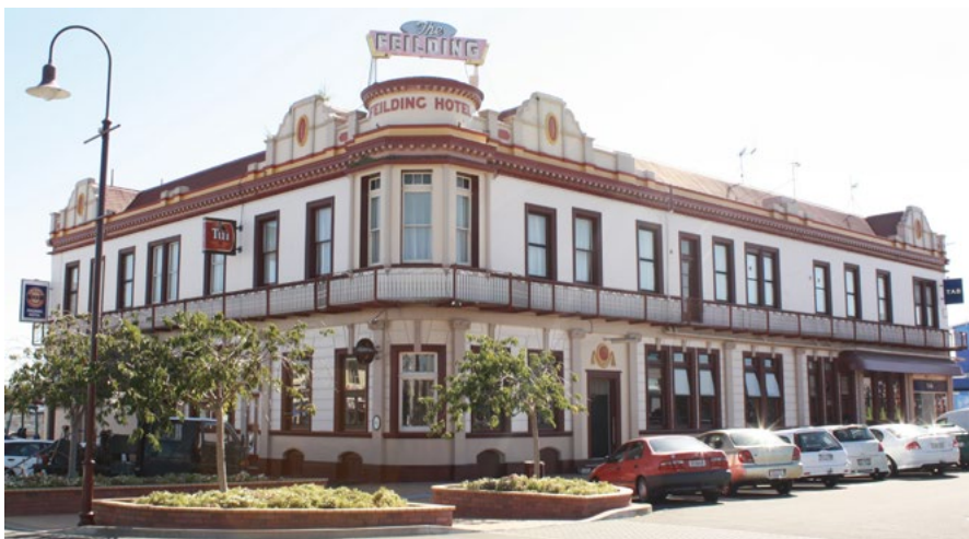
Feilding Hotel, 9 Manchester Square (constructed 1875-1910)
