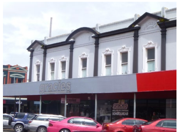
The good example above shows modulation created by a series of structural bays - highlighted in the dark colour in this instance. The bay 'modules' continue up the building to the top.
