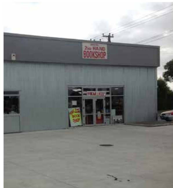
Refurbish / paint frontages to existing buildings
