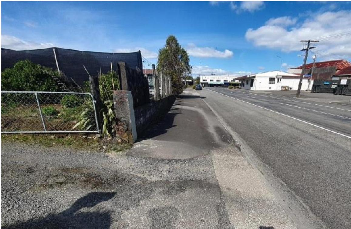
Example of poor condition Vehicle Entranceway that is affecting the condition of footpaths
