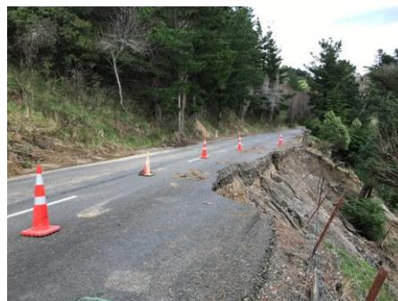
Road slumped into gully – Route 52
