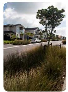
Planted Swales and open drains to manage stormwater on a localised level
