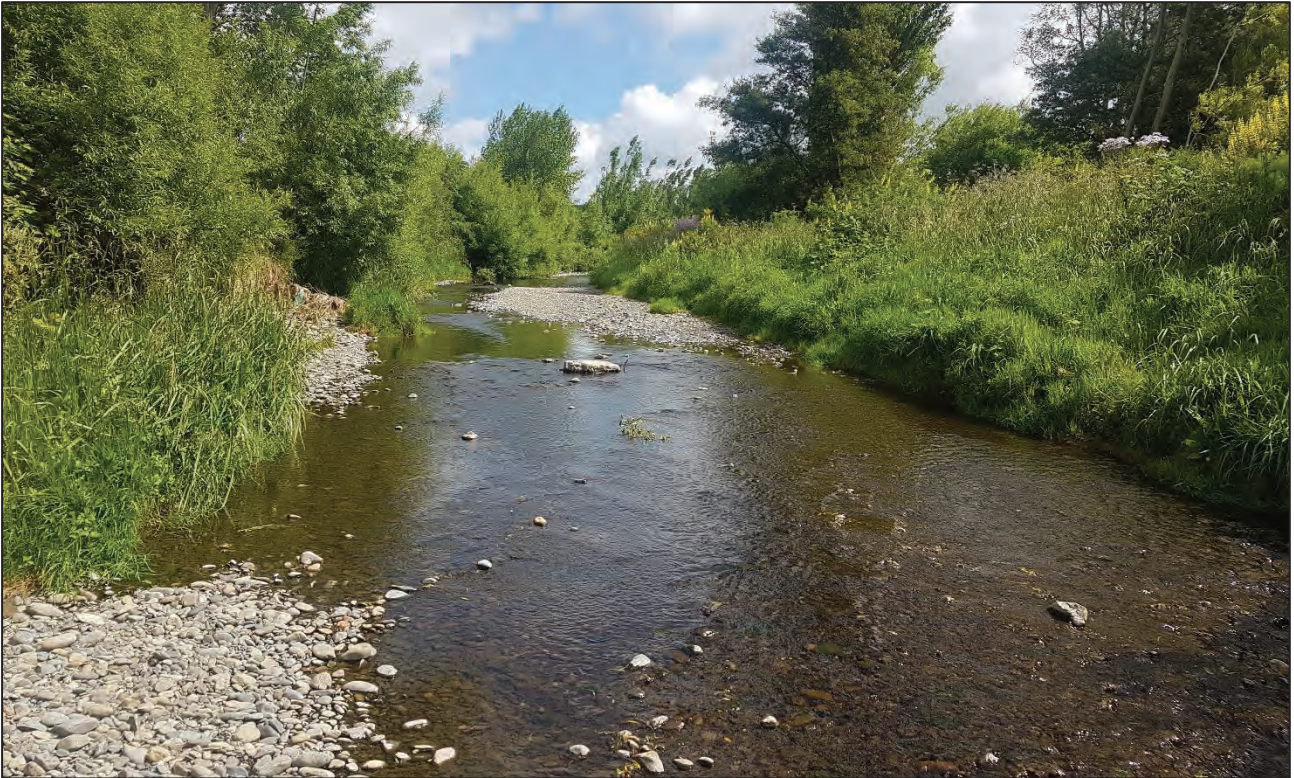
Figure 7: Looking up the Makino Stream at Roots Street.
