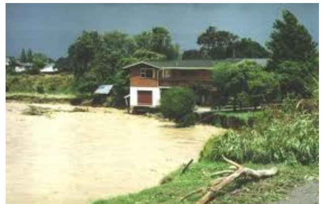
The Feilding town sits on a flood plain. It is important to plan new development to recognise hazards and to minimise the extent to which new development may exacerbate them
