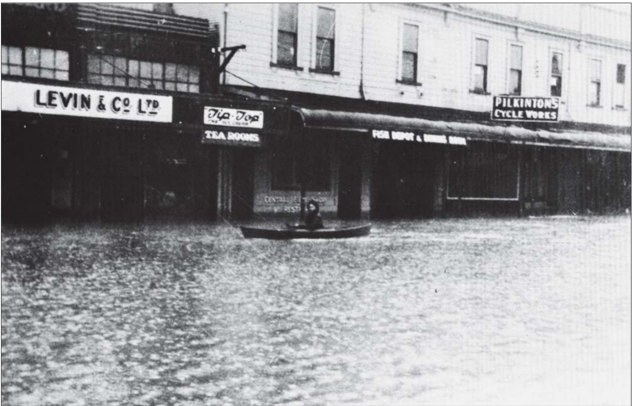
Figure 7: Flooding in the main street of Pahiataua – 24 June 1942
