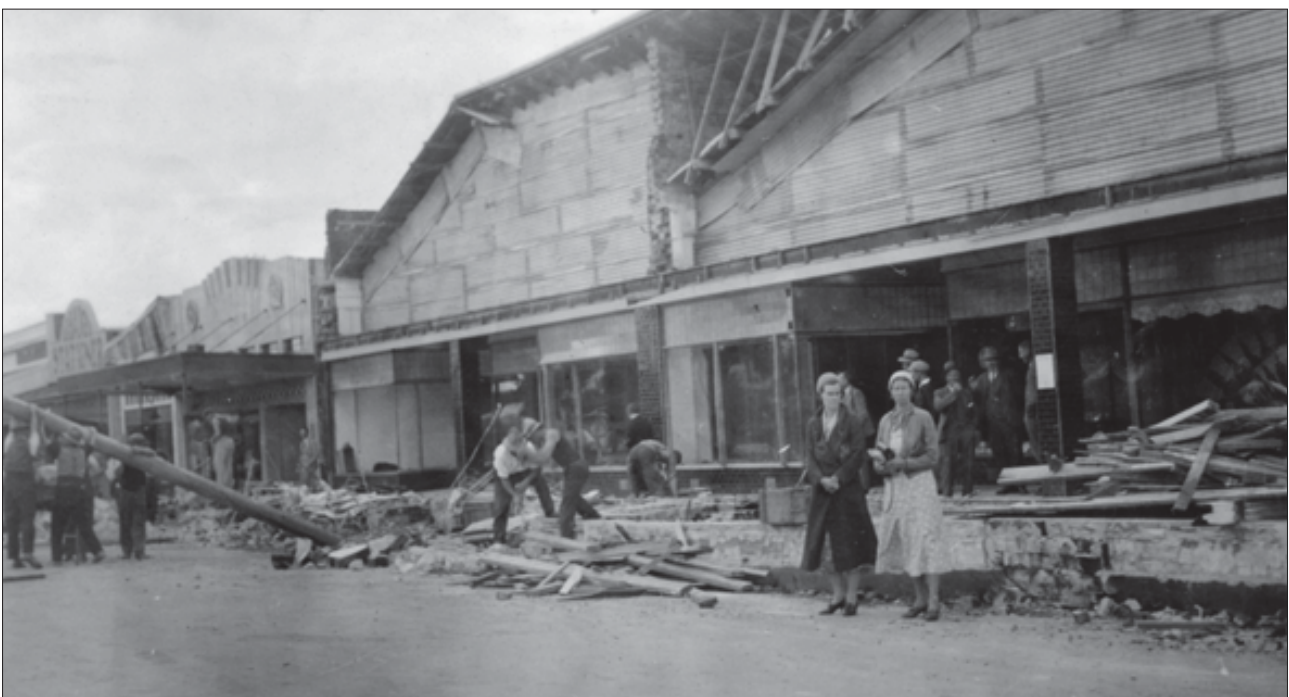
Figure 3: Workers remove debris from the Main Street of Pahiatua after the 1934 earthquake
