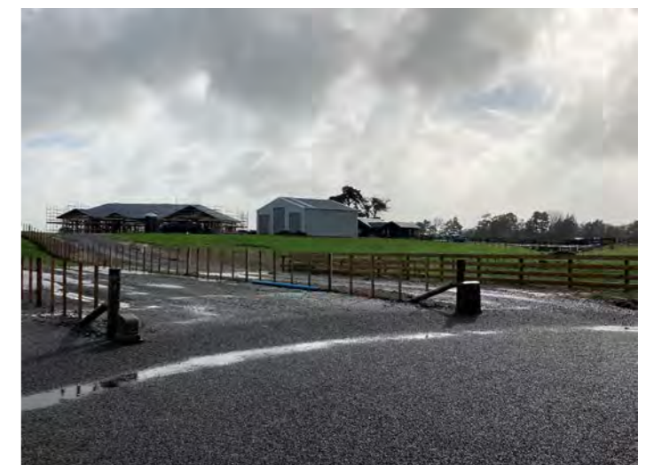
Neighbouring new properties under construction.
