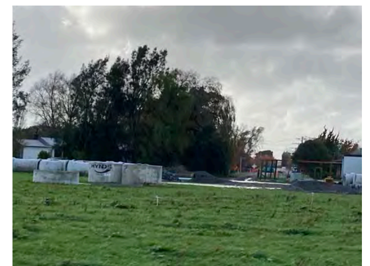
A stormwater infrastructure upgrade is currently underway at Trent Street.
