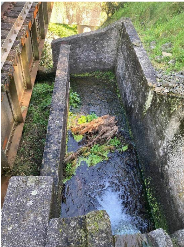
Figure 3.1: Photograph of drain north of rail bridge over Tamaki River
