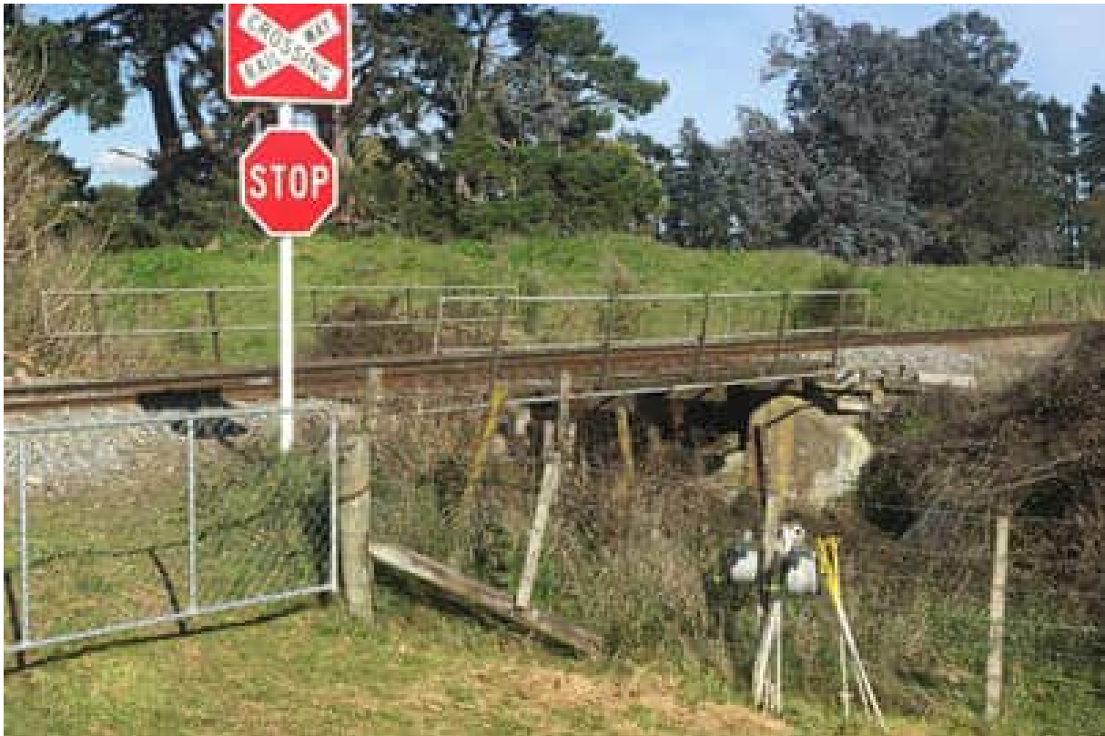
Figure 3.4: Photograph of rail bridge over Makirikiri Stream
