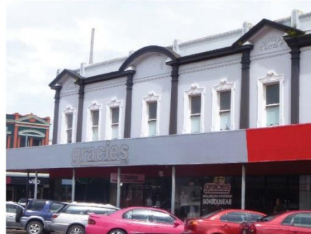
The good example above shows modulation created by a series of structural bays - highlighted in the dark colour in this instance. The bay 'modules' continue up the building to the top.
