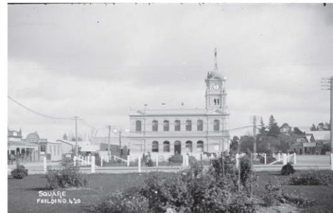
Photograph of Post Office (190P)
