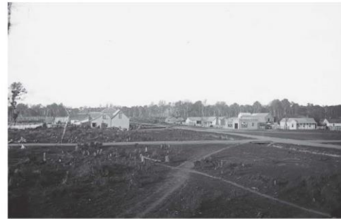
Photograph of the township of Feilding, Manchester Block, Manawatu (1878)
