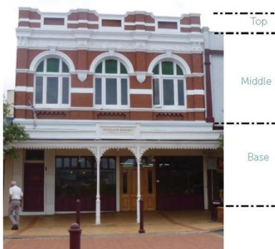
Vertical hierarchy of a base, middle and top is expressed in the size and shape of openings and balconies.
