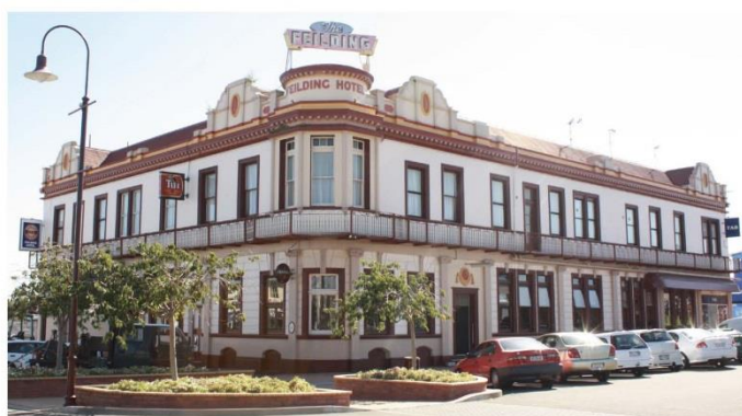
Feilding Hotel, 9 Manchester Square (constructed 1875-1910)
