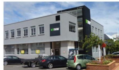
Photograph of 8 Manchester Street - (1949)
