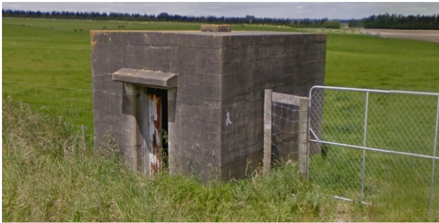
Figure 4 The small structure that contained the engine that powered the operations room (Source: Google Street View, November 2013)
