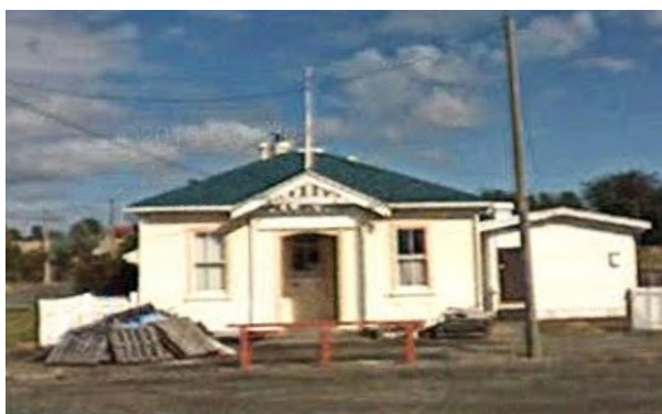
Figure 8 A Google Street View photo of the former post office in February 2008. The metal bike racks beneath the windows, were not yet back in place at this time.
