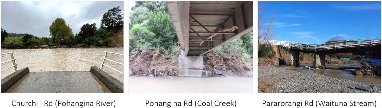
FIGURE 48: STRUCTURAL DAMAGE AND LOSS DUE TO ADVERSE WEATHER EVENTS
