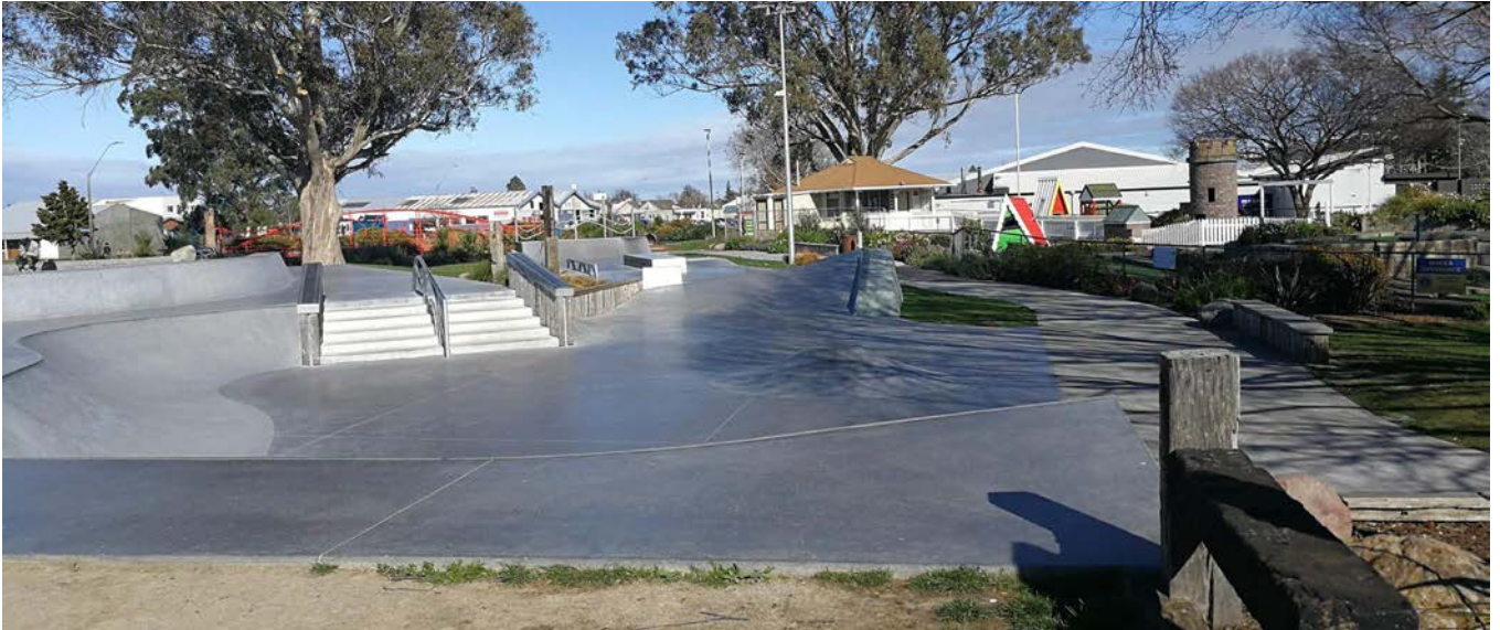
Photograph 1: Makino Skate Park from Church Street looking towards Manchester Street
