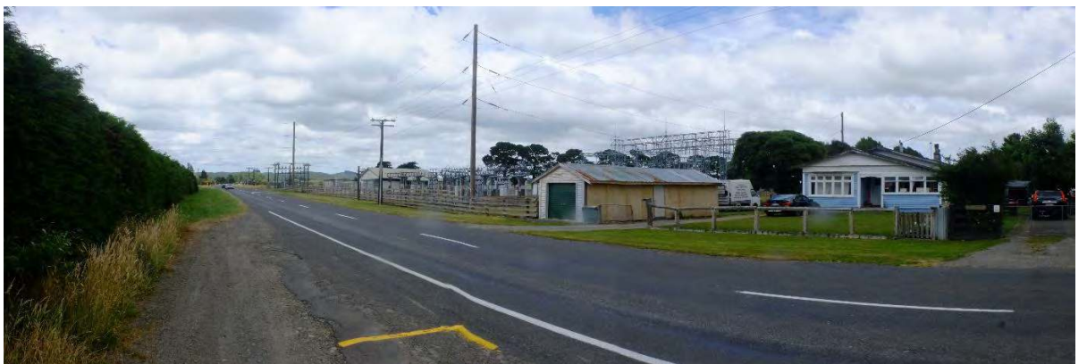
Fig 5: View of Mangamaire Substation from Tutaekara Road travelling east.
