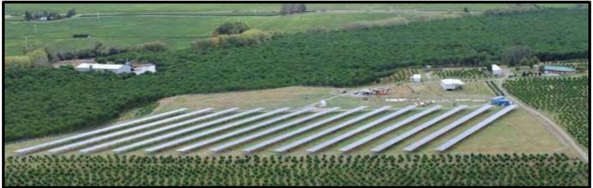
Figure 5: Example of a similar solar farm in Marlborough (Source: Appendix 2)
