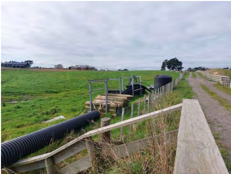
Plate D20: Looking east from southern boundary of the southwest lot. Note the stockpiles of drainage pipe and timber posts.
