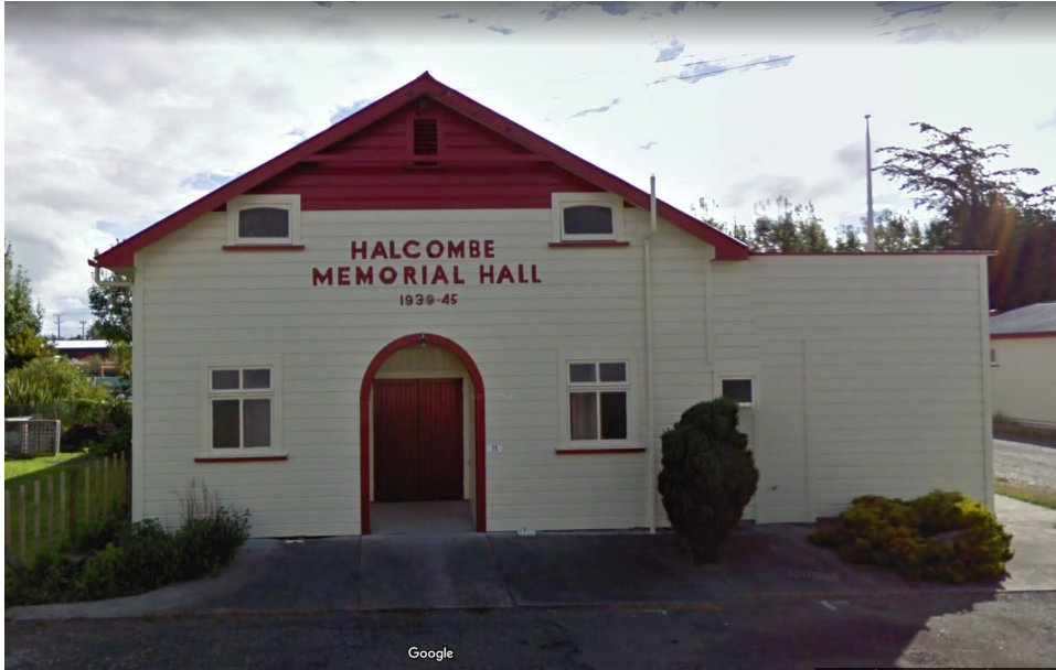
Figure 2 Halcombe Memorial Hall. Google Street View – February 2010
