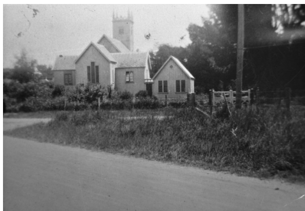
Figure 1 St. John's Church showing the attached Sunday School at right that was built in 1885 and burnt down in 1909.
