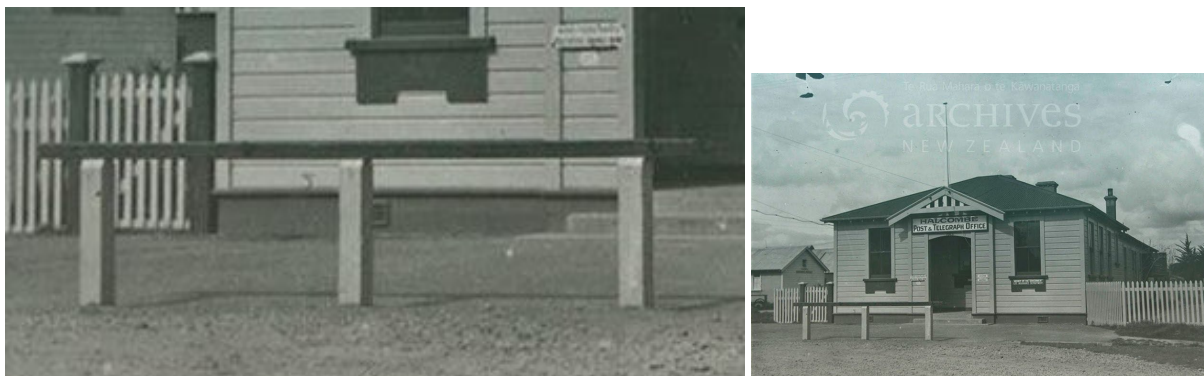
Figure 3 The hitching rail with a colour change, after both the building and rail have been painted. The building is known to have been painted in 1923. 1 There is no sign of the hitching hooks on this side of the structure. There is also no sign of a metal strap to hold the rail in place in this photo. (Source: Archives NZ, Wellington. Ref: R24136477 AAME 8106 W5603 276/1/H/24)
