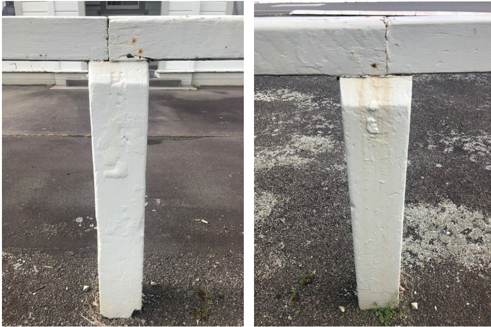
Figure 9 Both sides of the middle post – which shows a few interesting marks, causes of which may have included a metal strap over the top – as appears to have been present in the oldest known photo of the hitching rail. Whether or not both halves of the top rail are the originals, is not certain. (Photo: Rochelle Waugh, 26 September 2018)
