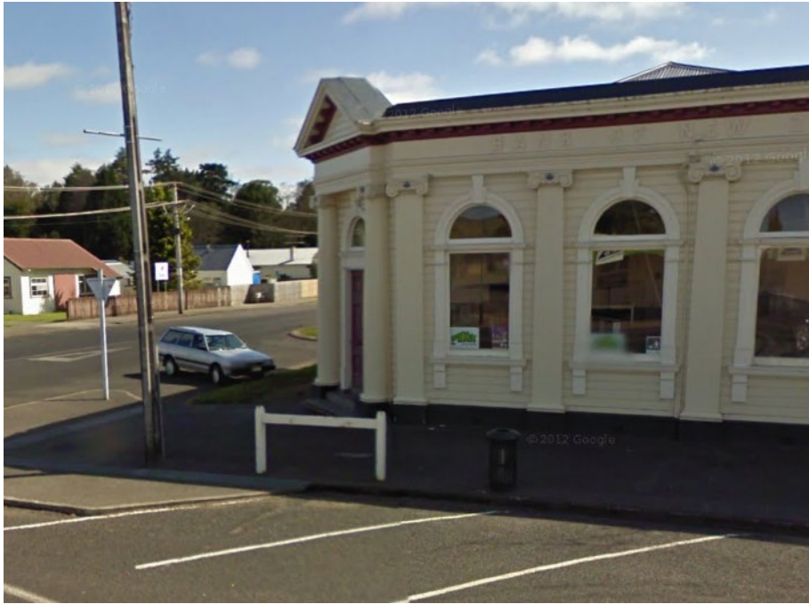
Figure 13 Raetihi Hitching Rail – Feb 2010. The hitching rings can just be seen on the rail in this photo. This hitching rail has a Category Two listing with Heritage New Zealand. (Google Street View)
