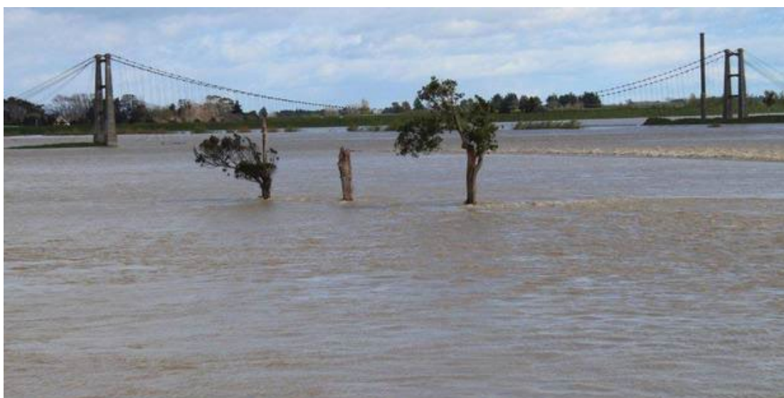
Figure 4 The Opiki Bridge, photographed by Alecia Rousseau from SH56, during a flood in September 2015 (Photo: NZ Herald , 24 September 2015: http://m.nzherald.co.nz/nz/news/article.cfm?c_id=1&objectid=11518335 )
