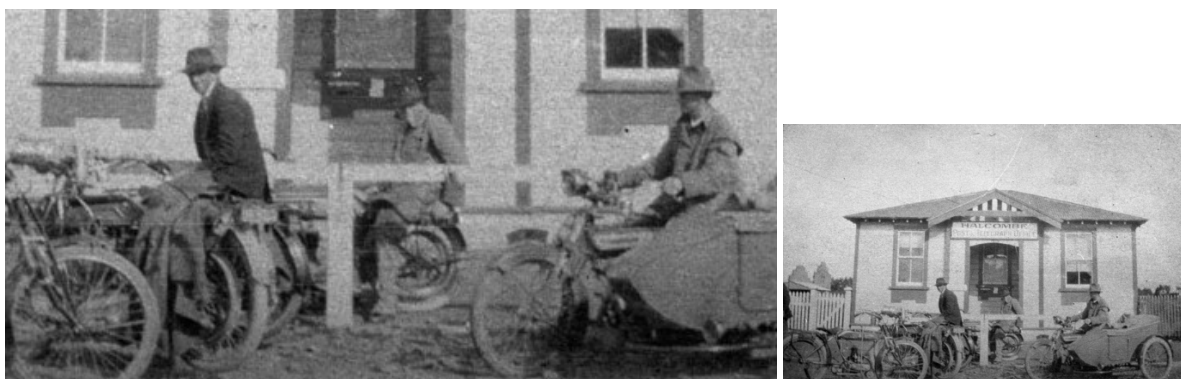
Figure 1 This is the earliest photo traced for this study that shows the hitching rail – which was installed in October 1914, thereby giving an earliest possible date. A noteworthy feature is that there appears to be a metal strap over the middle post in this photo. Such a strap would have served to (hopefully) hold the top rail in place when a misbehaving or startled horse pulled back on it. The other two posts are obscured. (Source: Mandahl Collection, Manawatu District Library http://feilding.recollect.co.nz/nodes/view/17871 )
