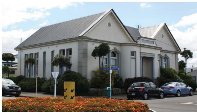
Feilding Community Centre, 21 Stafford Street (constructed 1910)
