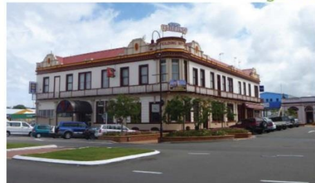
The facade of the Feilding Hotel is a good example as its openings are placed symmetrically, and as a corner building it has doors to both frontages
