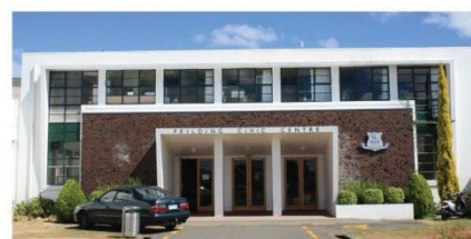
Photograph of Feilding Civic Centre, 84 Aorang Road (constructed 1957)
